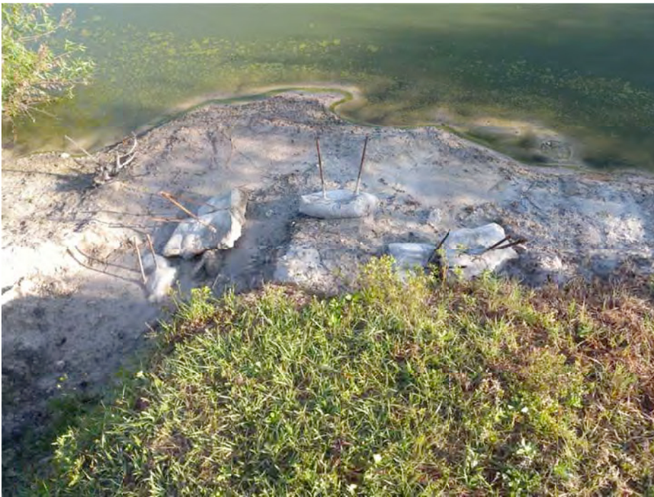
Pond 80 sand cement bags with riprap
